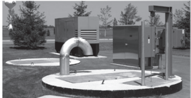
Lift Stations-New and Retro-fit Upgrades
