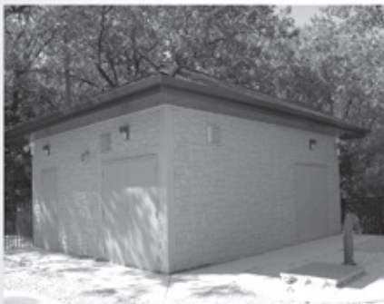
Housed Pump Systems
